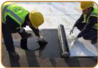
Apply Waterproofing Coatings & Membranes
