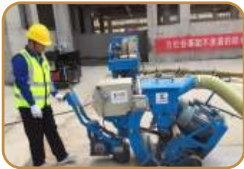
Substrate Shot Blasting Treatment
