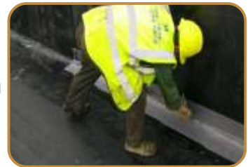
Reinforcement Treatment on Joints Parts
